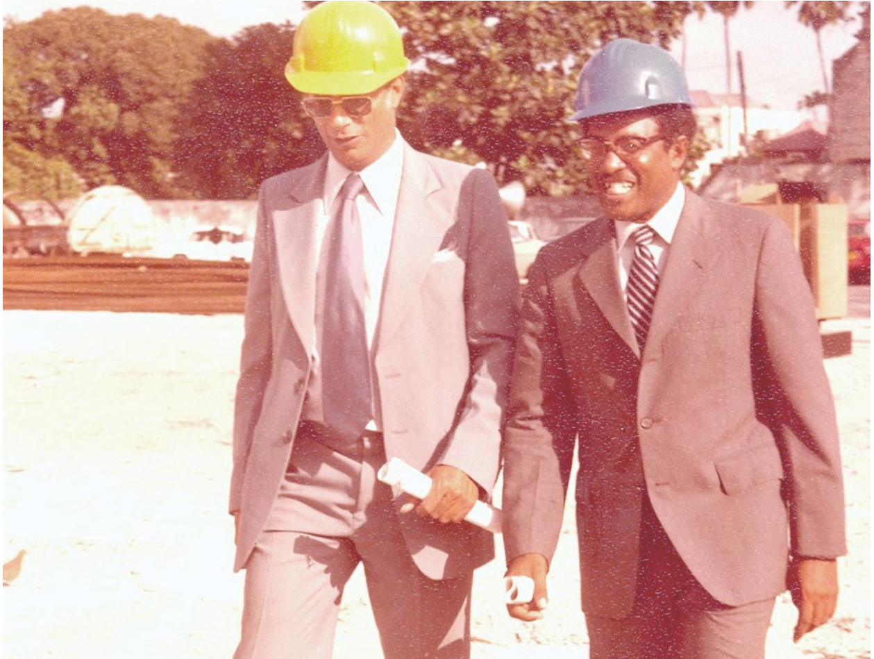
Dr. Blackman with then Prime Minister the Right Honourable J.M.G.M “Tom” Adams during the construction of the Central Bank of Barbados headquarters
